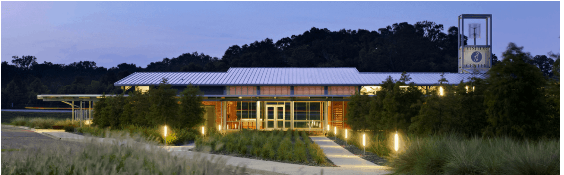
ST. LANDRY PARISH VISITOR INFORMATION CENTER
